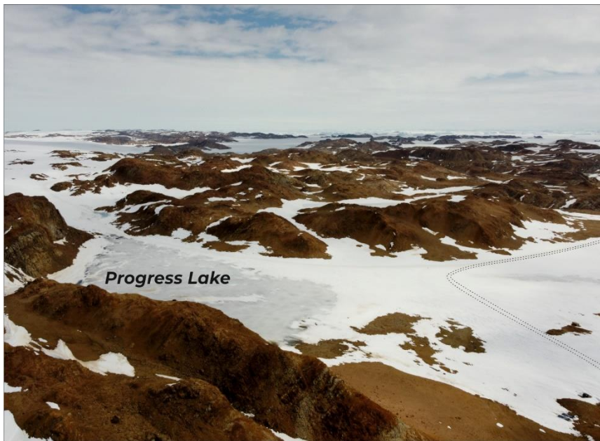
Fig. 21. View of the dam of Progress Lake on 13.12.2022
