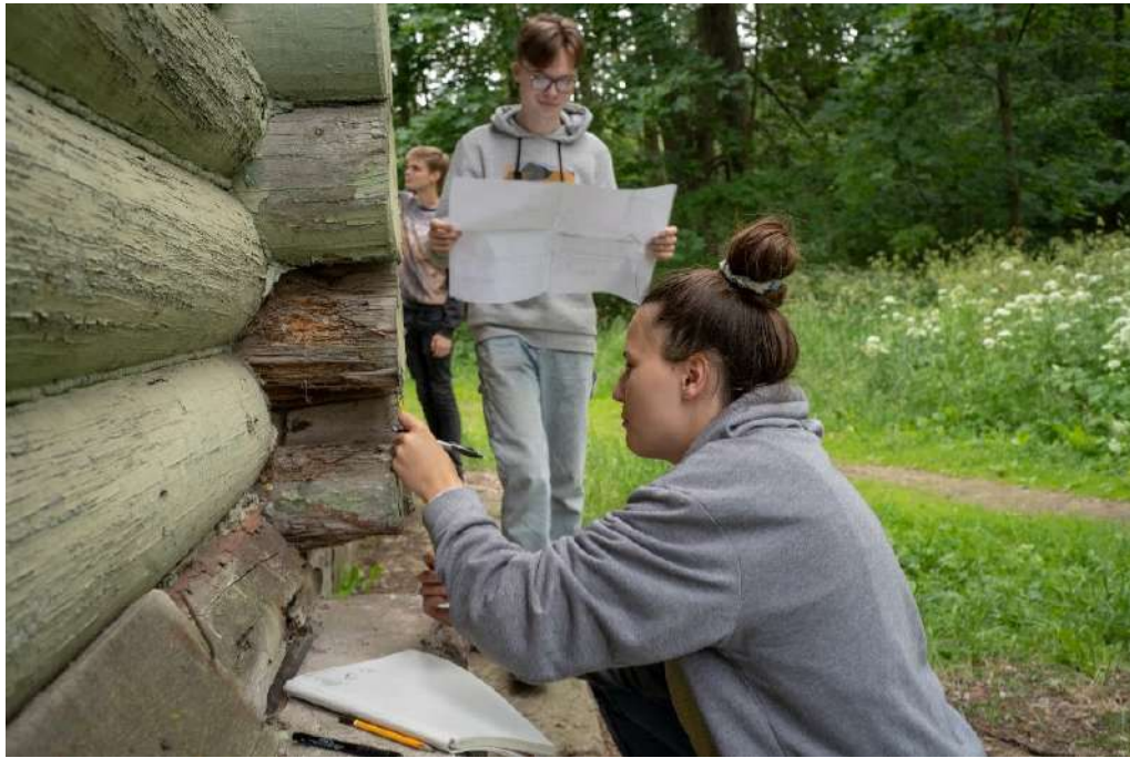
Field inspection of the Benois Dacha manually, July 2022.
